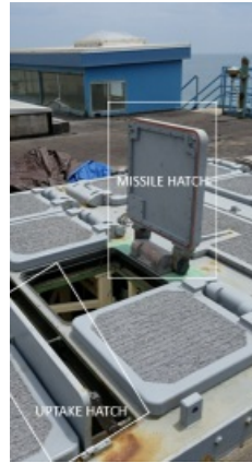
Image courtesy of Pacific Engineering Inc.
