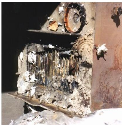
Close up of damaged incinerator
