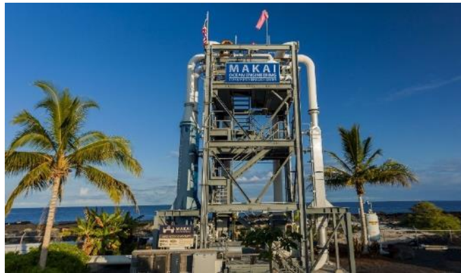
The Makai Ocean Energy Research Center is located in Kona
